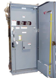
Load Break Switches (5KV and up)
